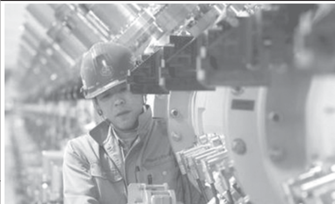
A worker works on a part of a 330 metres proton linear accelerator at a Japan Proton Accelerator Research Complex 'J-PARC' facility in Tokai village, about 130 km (81 miles) northeast of Tokyo on 16 May, 2006. —INTERNET
