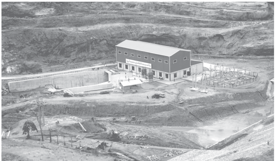
Yenwe hydel power station which can generate 125 million kilowatts hours per year. —MNA
