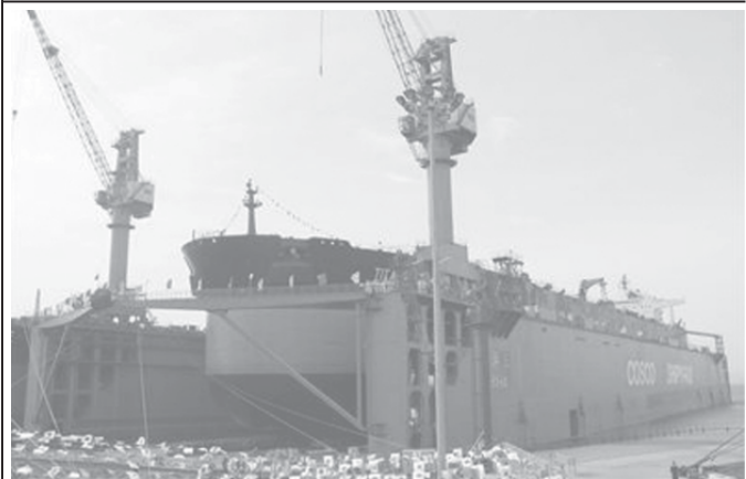
A 300,000-ton floating dock, the largest of its kind in the world, went into production on 10 May, 2006 in northeast China's coastal city of Dalian. Developed and built by the COSCO Shipyard Group Co, Ltd, the dock, which is 340 metres long, 76 metres wide and 27 metres deep, is capable of repairing 300,000-ton crude oil carriers, bulk freighters, and container ships, and rebuilding or converting other large watercraft.—INTERNET
