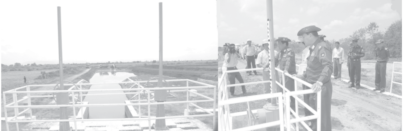
Lt-Gen Ye Myint of Ministry of Defence inspects the canal of Thittatkon Diversion Dam in Myitha Township. — MNA
