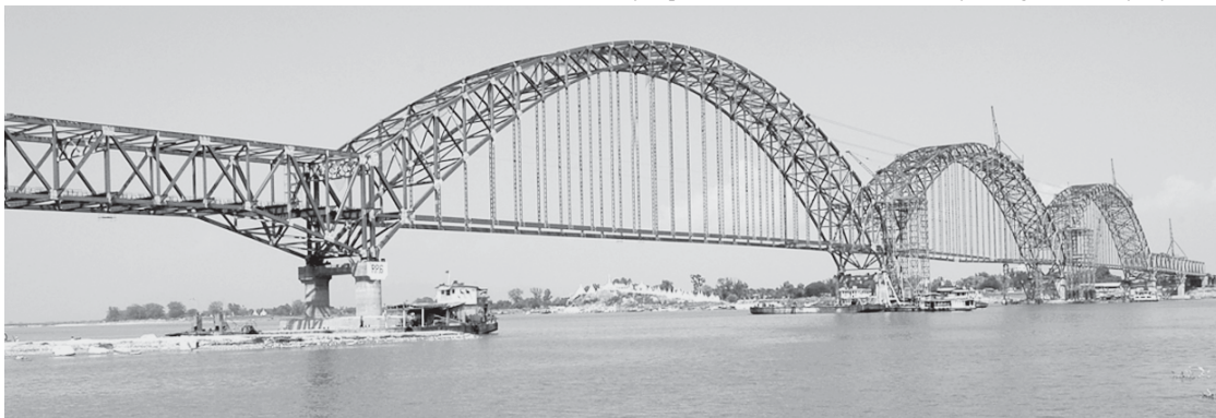
Ayeyawady Bridge (Yadanabon) under construction. — MNA
