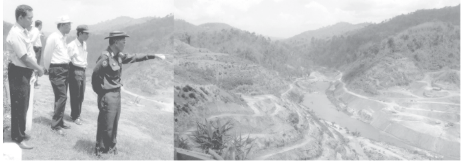
Minister Maj-Gen Tin Htut inspects Ahtet Paunglong hydel power project. —ELECTRIC POWER
