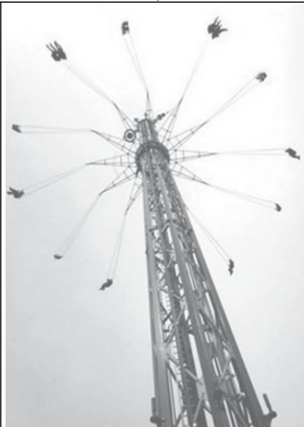
The first riders on what is billed as the world's tallest merry-go-round spin on 1 May, 2006 at Tivoli Gardens in Copenhagen, Denmark. The Star Flyer tops out at 70 metres (230 feet) above the ground and swings at speeds of up to 70 kph (43 mph). —INTERNET
