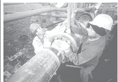
Two men work on a pipeline recently. A proposed gas pipeline from Iran to Pakistan and India will not be affected if the United Nations imposes sanctions on Teheran over its controversial nuclear programme, an Iranian minister has said.
