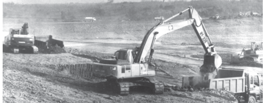
The construction site of Ma Mya Dam Project being implemented by Construction (9) of the Irrigation Department under the Ministry of Agriculture and Irrigation.
