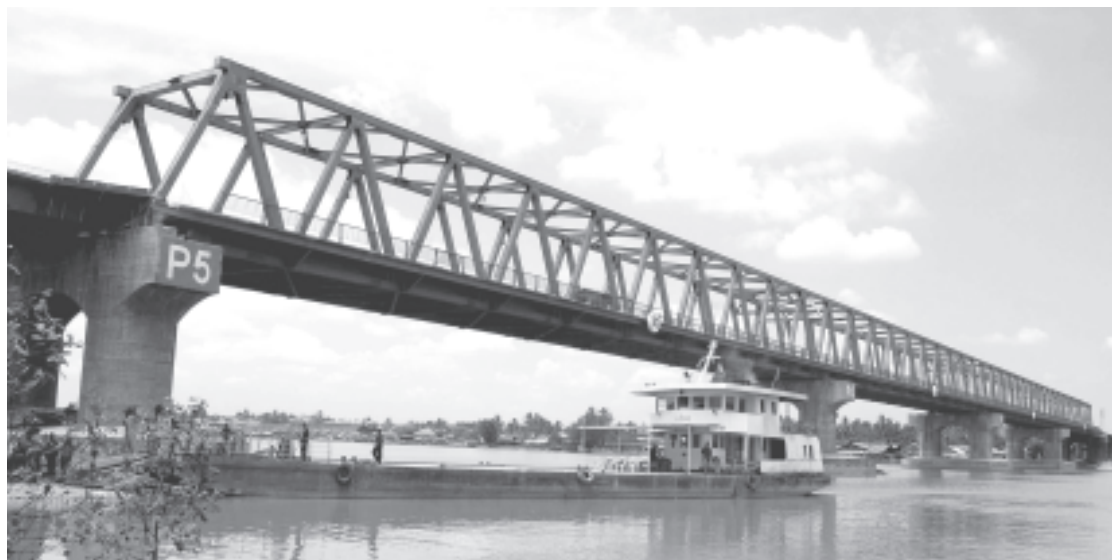
Construction of Pyapon Bridge in progress. — MNA
