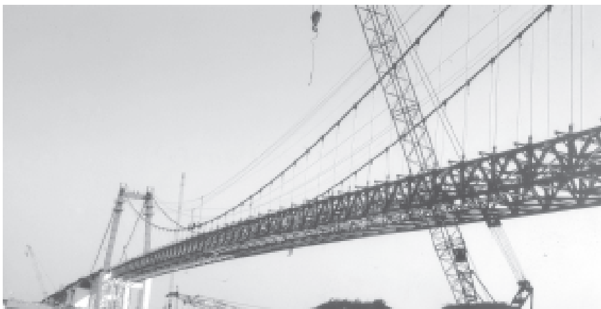
The photo shows the Twantay Bridge, which is nearing completion.
