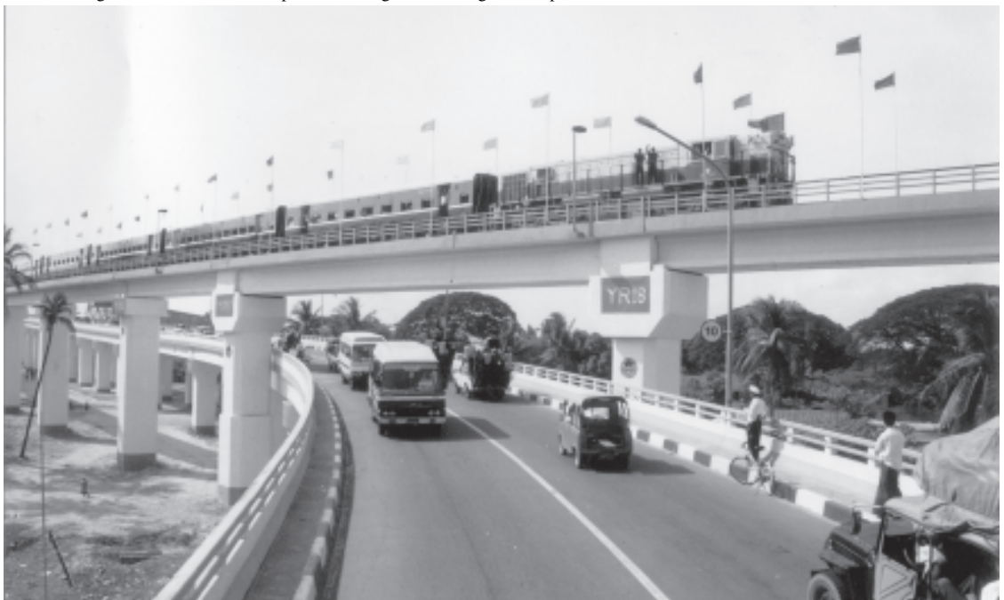
A train crossing over Thanlwin Bridge (Mawlamyine) at the opening day of the rail bridge. — MNA
