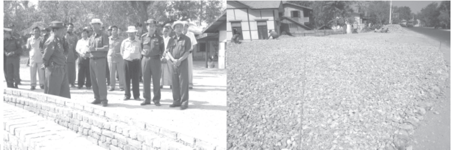
State Peace and Development Council Member Lt-Gen Ye Myint of Ministry of Defence inspects construction of approach road to Ayeyawady Bridge (Yadanabon). — MNA
