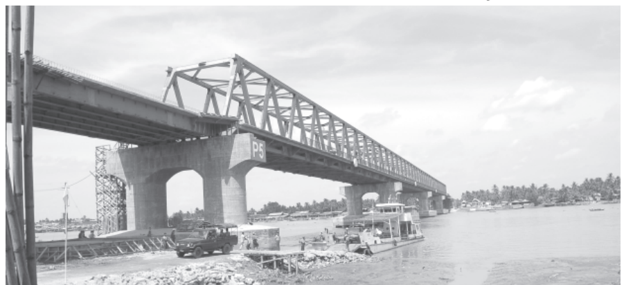
The photo shows Pyapon Bridge under construction. — MNA
