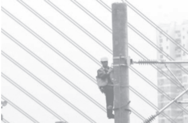
A worker repairs the power lines near the railway station in Shanghai on 4 April, 2006. A new high-speed rail line linking the Chinese cities of Beijing and Shanghai will cost more than $16 billion and will be open to private and foreign investment, a newspaper said on Tuesday.—INTERNET
