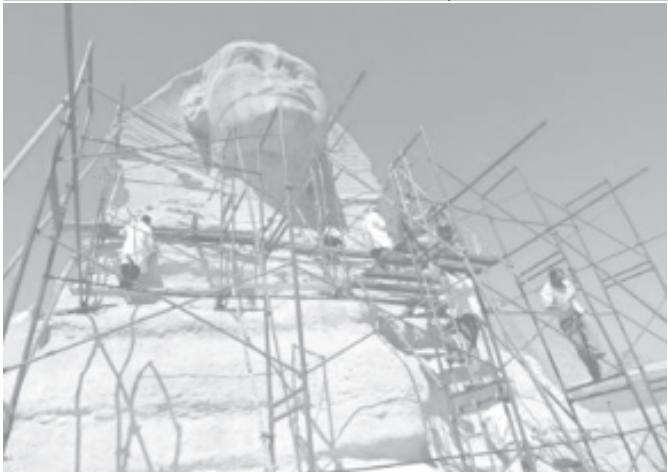
Workers carry out restoration works on the Great Sphinx of Giza in Egypt, on 3 April, 2006. The restoration effort will concentrate on the neck and chest of the Sphinx which have been eroded over time by the desert winds.—INTERNET
