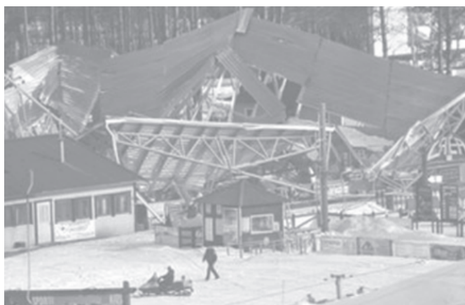
A skating rink with a collapsed roof at Okhta Park, on the outskirts of St Petersburg, Russia, on 31 March, 2006. Two children were injured Friday when the roof of a skating rink collapsed possibly due to heavy snow accumulation.—INTERNET
