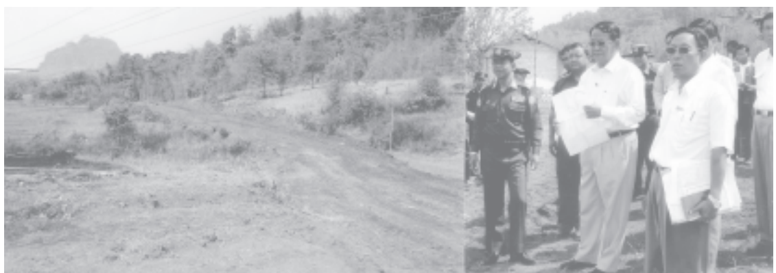
Commander of Eastern Command Maj-Gen Ye Myint and Minister for Industry-1 U Aung Thaung inspect construction of the axis of Tonhon-Pinlaung Road. — INDUSTRY-1
