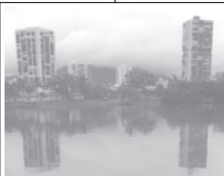
A temporary sewage line leads directly into the Ala Wai Canal just behind Waikiki on 29 March, 2006 in Honolulu, Hawaii. A sewage-line leak in Waikiki forced the City of Honolulu to divert millions of gallons of raw sewage into the Ala Wai Canal, which empties directly into Oahu's South Shore, turning the usual greenish-blue water into a brown murky colour. High levels of bacteria have been detected in several of Waikiki's most famous beaches causing the City's Health Department to post warning signs on the beaches warning swimmers and waders of contamination in the water. —INTERNET
