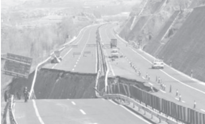
A cave-in on the Shouyang section of an expressway linking the capitals of Hebei and Shanxi provinces in North China brought traffic to a standstill, on 28 March, 2006.—INTERNET
