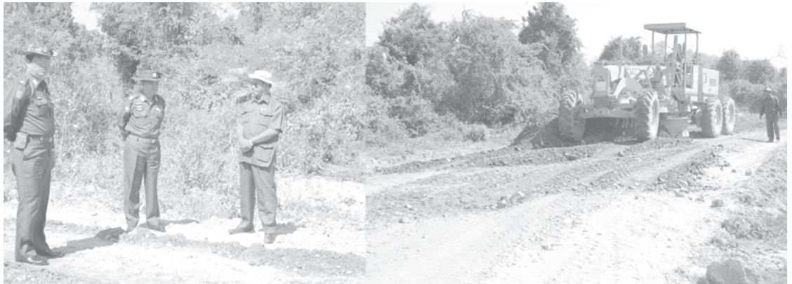
Lt-Gen Khin Maung Than inspects construction of Pathein-Mawtin Road. — MNA
