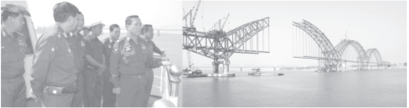
Prime Minister General Soe Win inspects construction of approach bridges and main structure of Ayeyawady Bridge (Yadanabon). — MNA
