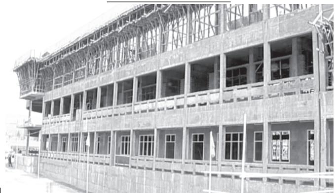
The three-storey main building of Government Technical College (Lashio).—MNA
