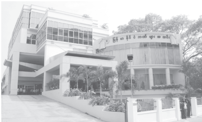
Newly opened building of Myanmar Banks Association.
