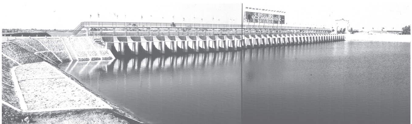
Yin Nyein Sluice Gate in Paung Township, Mon State, is serving the regional as well as national interest. — MNA
