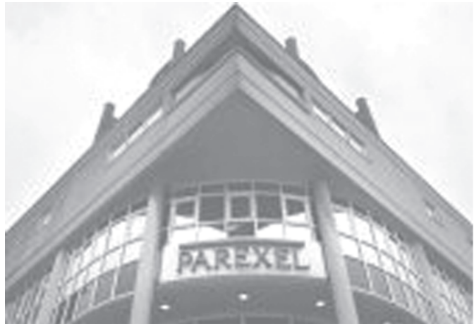
The headquarters of Parexel drug company are seen in Uxbridge on 16 March, 2006 west of London, England. Six volunteers remain in hospital after becoming ill during the first human trials of the TGN1412 drug made by Parexel.—INTERNET
