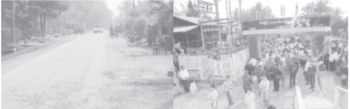
Lt-Gen Ye Myint inspects the road and Myolechaung Bridge in Htigyaing Township. — MNA
