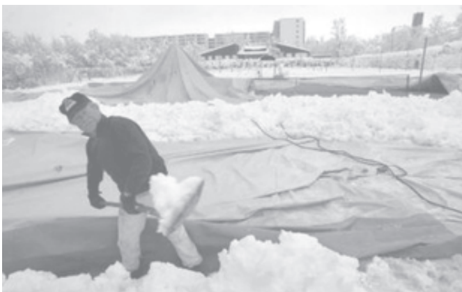
A volunteer shovels snow from the collapsed plastic roof of a tennis centre in Munich on 5 March, 2006. The roof collapsed under the weight of heavy snow. In southern Germany, snow fall has disrupted local transport and domestic flights. —INTERNET
