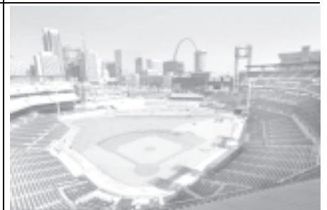
The view from the upper deck of the New Busch Stadium under construction in St. Louis, Missouri, on 3 March, 2006. Most of the stadium, with the exception of a few thousand seats, is projected to be ready for the St Louis Cardinals' home opener scheduled for 10 April, 2006 against the Milwaukee Brewers. —INTERNET
