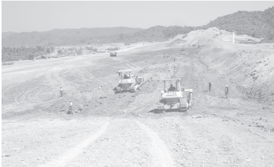
Construction site of Kataik Dam in Paung Township. — MNA
