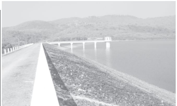
Wapah Dam in Thaton in progress. — MNA
