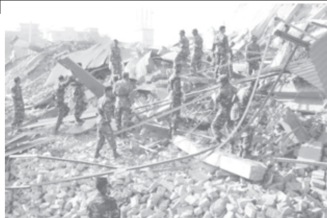
Army soldiers remove the debris of the garment factory that collapsed in Dhaka on 25 Feb, 2006. —INTERNET
