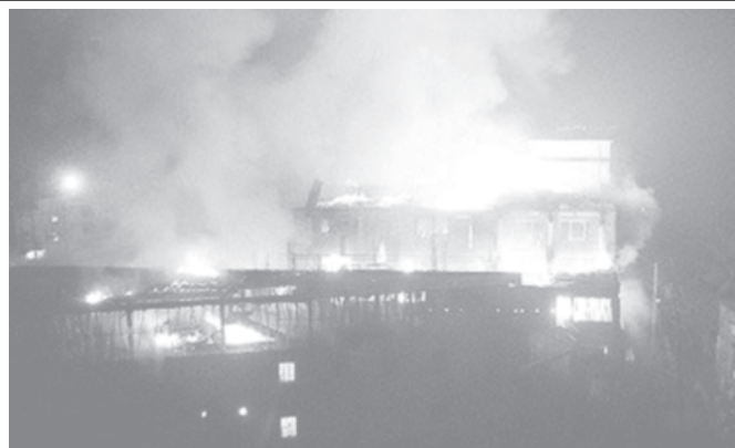
A fire engulfs a textile factory, at the Kalurghat area of Bangladesh's port city of Chittagong.—INTERNET
