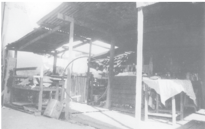
Kitchen of a restaurant being seen after the bomb blast. — MNA
