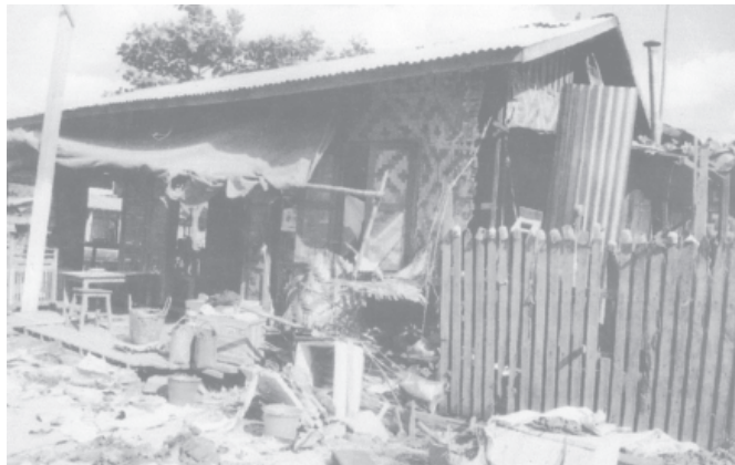
Kitchen of a tea-shop being damaged because of the bomb blast. — MNA
