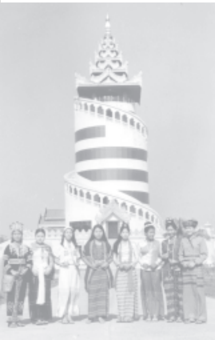
Nanmyint Tower at Union National Races Village.
