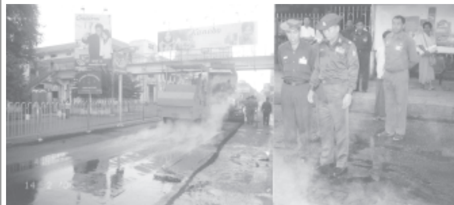
Mayor Brig-Gen Aung Thein Linn inspects tarmacking of Bogyoke Aung San Street in Pabedan Township on 14-2-2006. — YCDC
