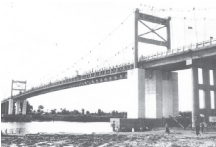
Zarthabyin Bridge across Gyaing River on Mawlamyine-Zarthabyin-Eindu-Hpa-an Road in Kayin State.
