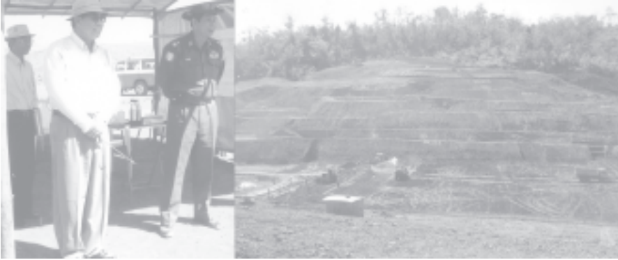
Minister for Agriculture and Irrigation Maj-Gen Htay Oo oversees progress in construction of Maday Dam in Kanma Township. — A&I
