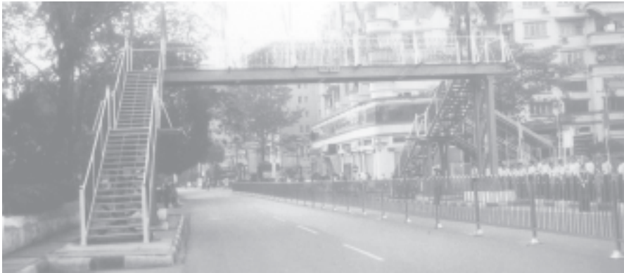
Dagon overpass at Alanpya Pagoda Road in Dagon Township. — MNA
