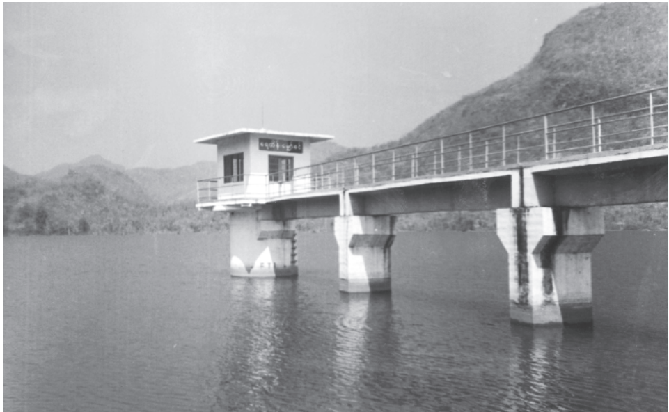
The Loinanpha Dam built in Dimawhso Township, Kayah State.
