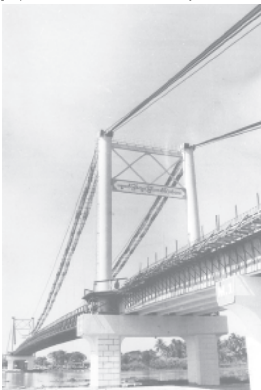
Pammawady River Crossing Bridge (Myinkaseik) linking Myaungmya and Pathein.
