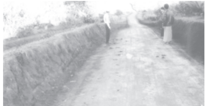
Nawngkhio-Thanhayaaye rural road in Nawngkhio Township, Shan State (North) on 3 January 2006.
