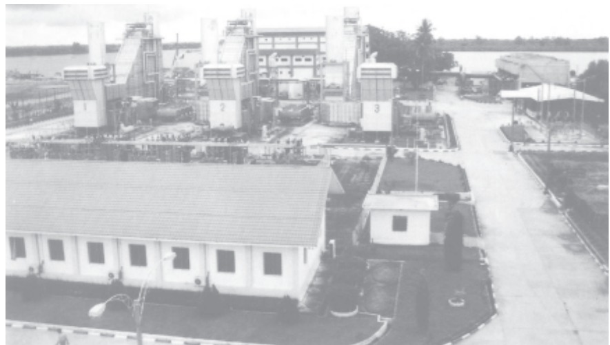
Waste heat recovery power plant in Ahlon Township, Yangon Division.
