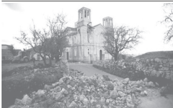
A damaged church is seen in the village of Mitata, on the Greek island of Kithira on 9 Jan, 2006, following Sunday's magnitude-6.9 undersea earthquake. The quake struck between Kithira and Crete, southern Greece. —INTERNET
