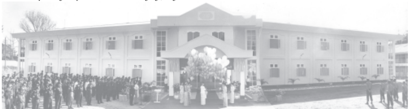
A new two-storey Khwa Nyo hall in CICS (Phaunggyi).—MNA
