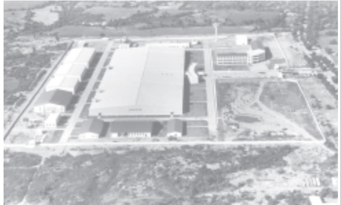
An aerial view of Myanmar Textile Factory (Salinyi) in Salinyi Township, Monywa District, Sagaing Division.
