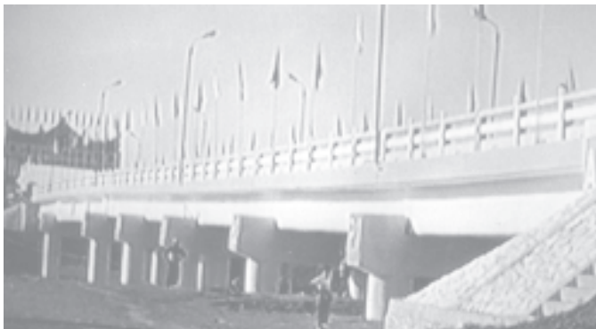
Newly-inaugurated Panlaung Bridge in Singaing Township.— MNA
