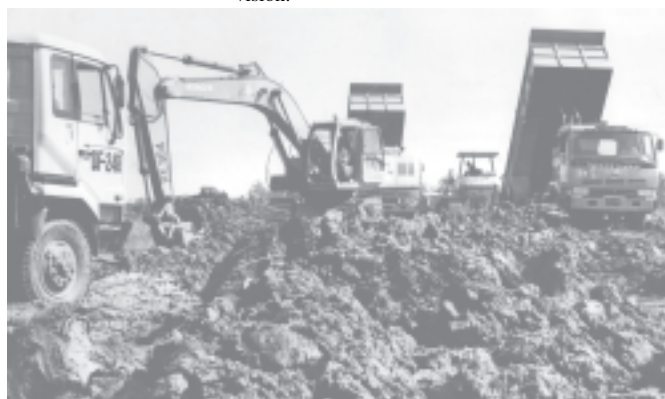
Heavy machinery being operated for construction of the main embankment of Kayan Sluice Gate Project.
