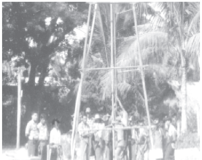
Photo shows sinking of a tubewell in Ywama Village, Kantbalu Township, Sagaing Division. — PBANRDA
