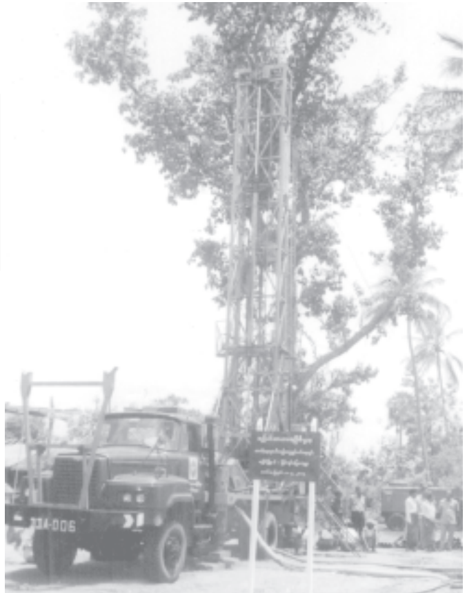
Tubewells are being sunk to supply water to the people living in Myitkyin Model Village in Mahlaing Township, Mandalay Division. — PBANRDA
