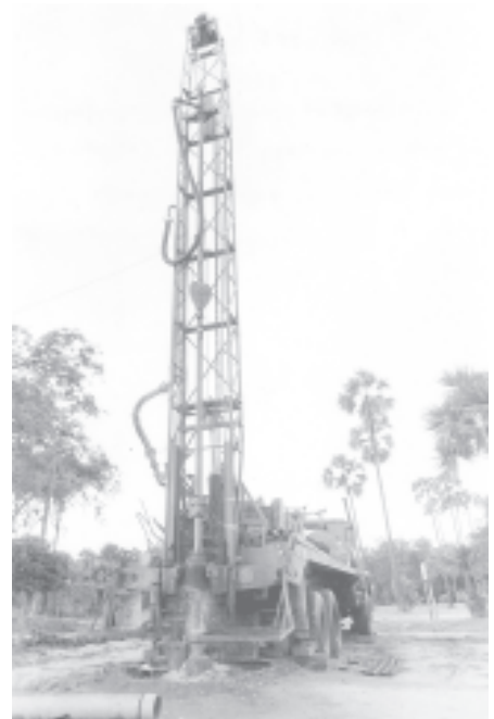
A tube well being sunk for rural water supply in arid region in central part of Myanmar.
