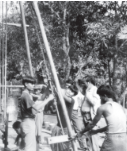
A tubewell is sunk to supply potable water to rural people living in Indaw, Sagaing Division. — KYEMON
