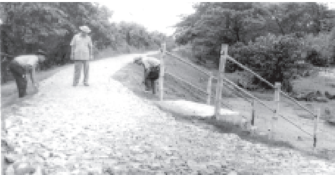
New roads are being built in rural areas for better transportation. The photo shows gravelling of roads in Thonekhwayun village, Maubin Township, Ayeyawady Division. PBANRDA
