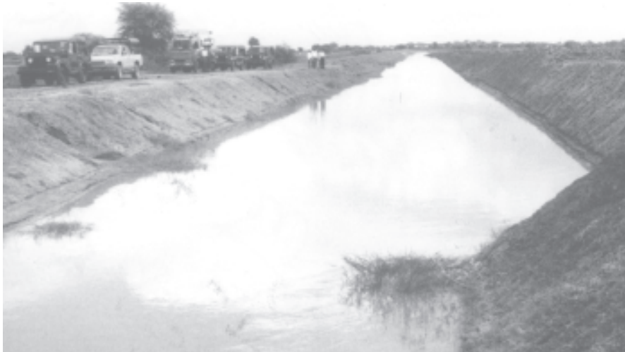
Thittetkon Diversion Weir in Myittha Township, Mandalay Division, constructed by the people and the Tatmadaw.
