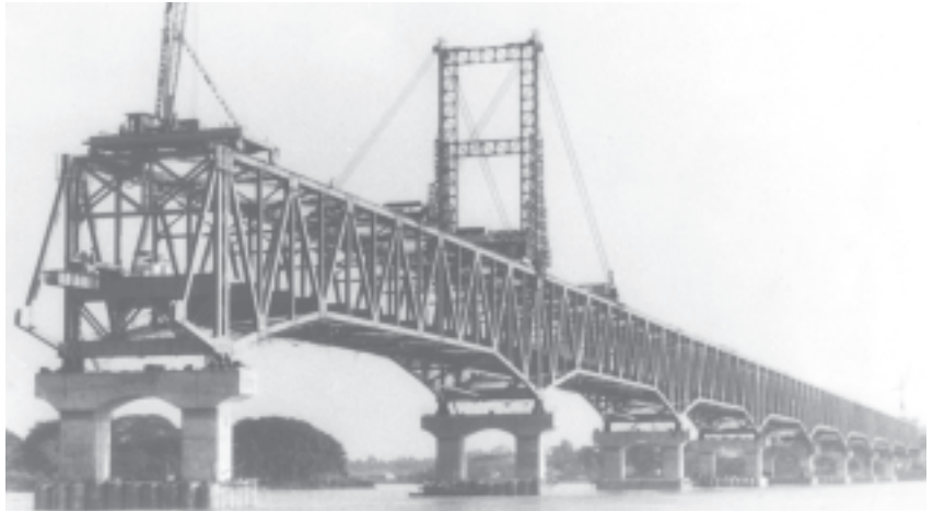
Thanlwin Bridge (Mawlamyine) under construction on Yangon-Mawlamyine-Myeik-Kawthoung road. On completion, it will be the longest bridge in Myanmar with 26,466 feet in length.
