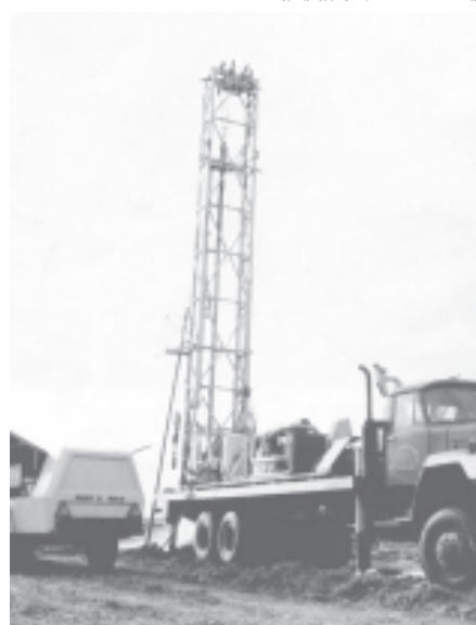
Drilling machines at work to get potable water for local people in Kantha village, Budalin Township, Sagaing Division.
