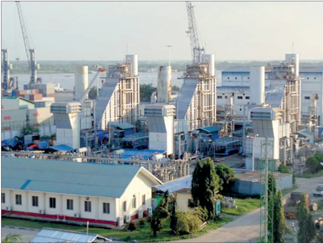
Ahlon Natural Gas Power Station . MOEE
